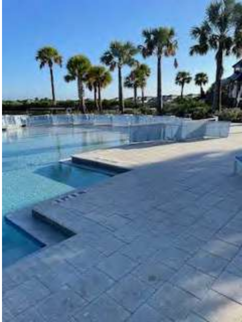
East side of the pool area near the zero-entry looks good other than the loungers laying on their sides which does not prevent any ducks from entering the pool area. Palm trees need trimming.
