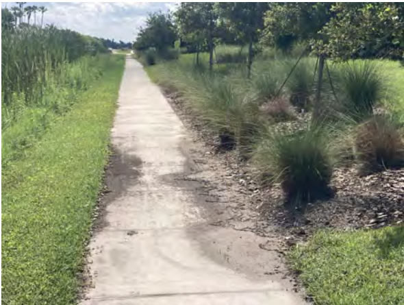
Sidewalk On 11th Street 1
